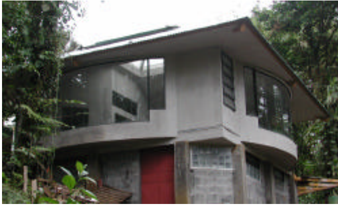
Construction of the café in July 2003
